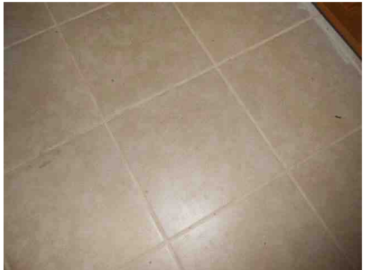
new kitchen tile
