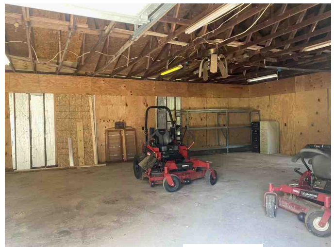
INTERIOR OF DETACHED SHOP
